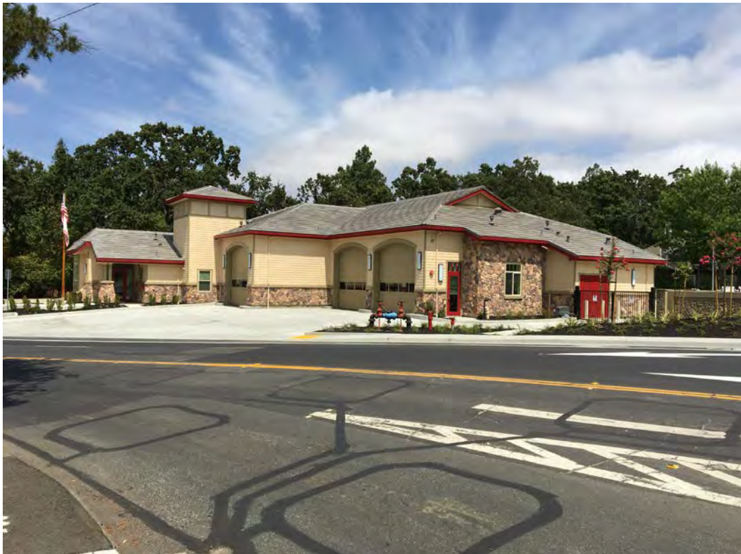
SW CORNER OF STATION 32
