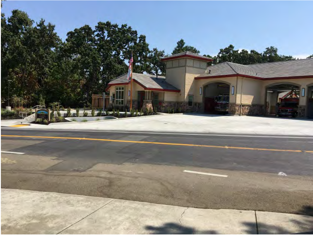
WEST SIDE OF STATION 32 FROM MIRANDA AVE
