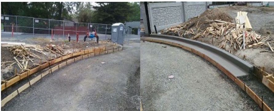
Curbs and gutter poured through middle drive lane
