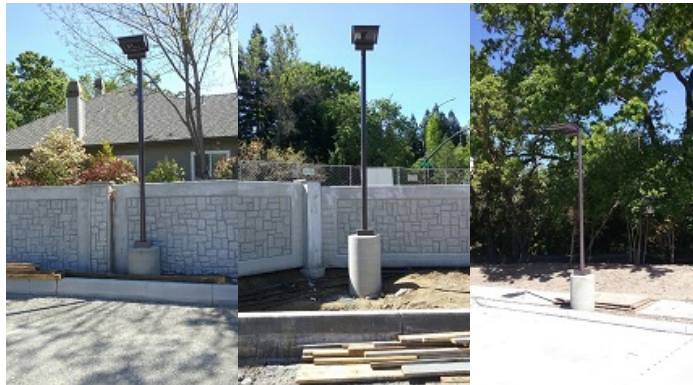
Light poles installation
