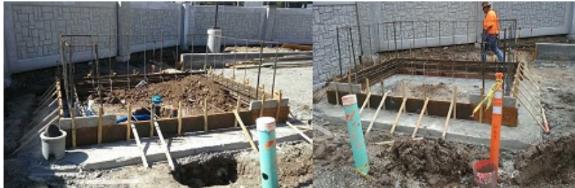
Trash enclosure footing and concrete pad
