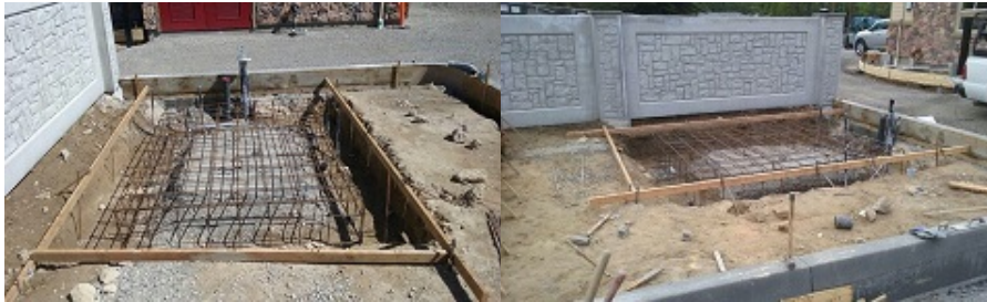
Foundation w/rebar footing and forms- aboveground fuel tank
