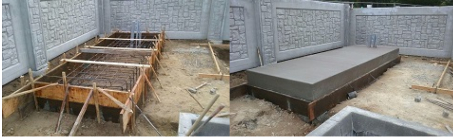
Emergency Generator form w/rebar and concrete pad
