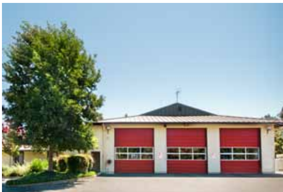
Station 34 12599 Alcosta Boulevard San Ramon
