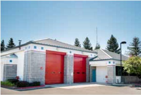
Station 38 1600 Bollinger Canyon Road San Ramon
