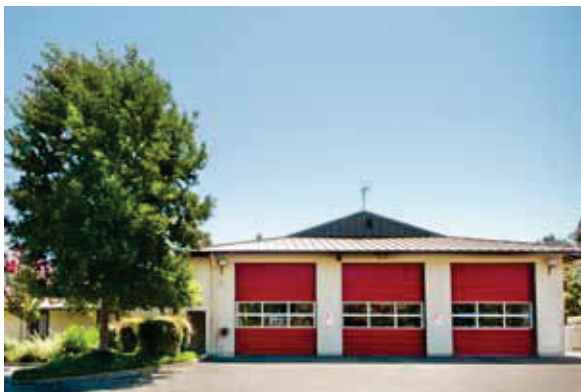
Station 34 12599 Alcosta Boulevard San Ramon
