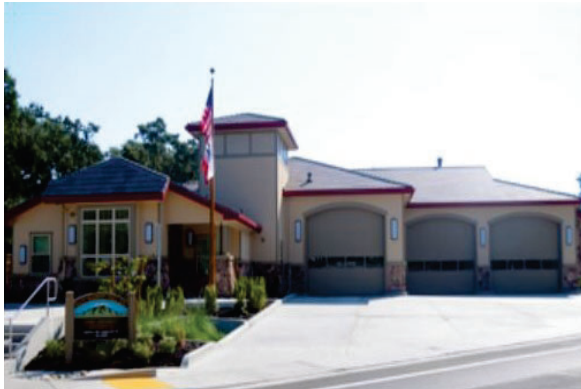
Station 32 2100 Stone Valley Road Alamo
