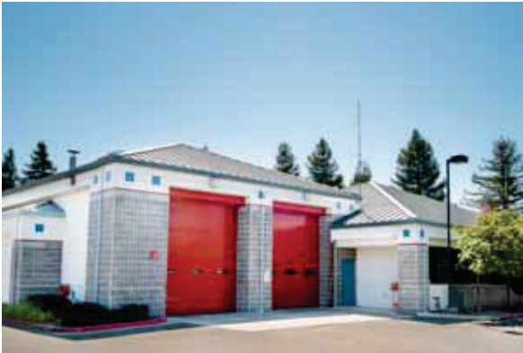
Station 38 1600 Bollinger Canyon Road San Ramon
