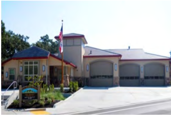
Station 32 2100 Stone Valley Road Alamo
