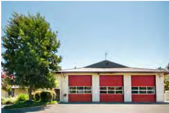
Station 34 12599 Alcosta Boulevard San Ramon
