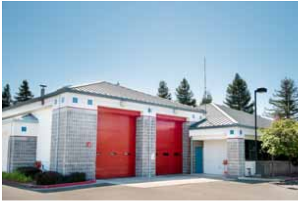
Station 38 1600 Bollinger Canyon Road San Ramon
