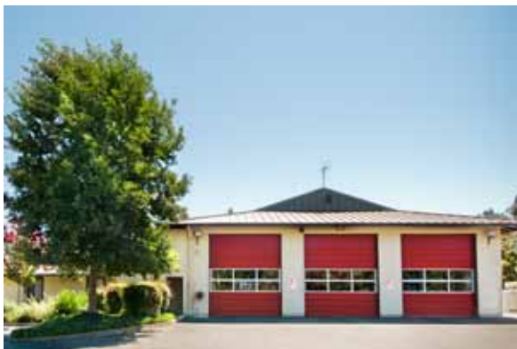
Station 34 12599 Alcosta Boulevard San Ramon
