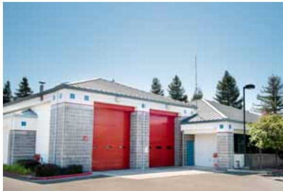
Station 38 1600 Bollinger Canyon Road San Ramon
