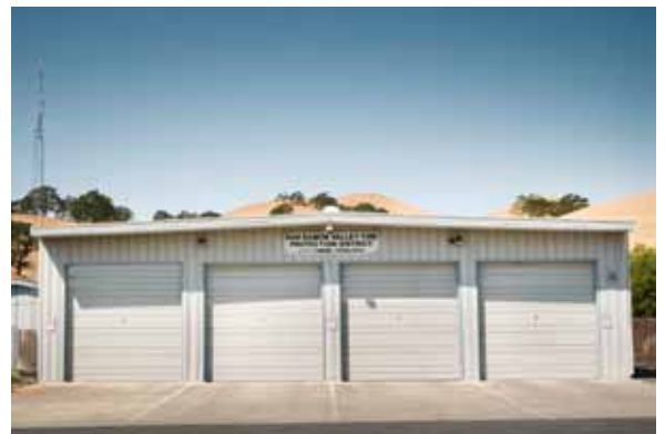
Training 6100 Camino Tassajara Road Tassajara
