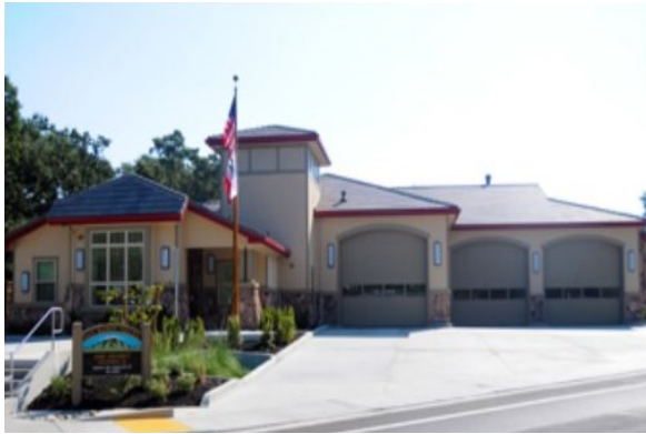
Station 32 2100 Stone Valley Road Alamo
