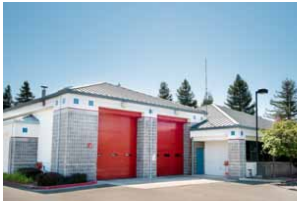
Station 38 1600 Bollinger Canyon Road San Ramon
