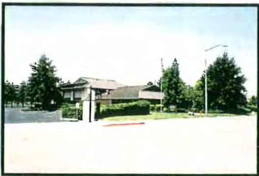
Station 34 12599 Alcosta Blvd., San Ramon
