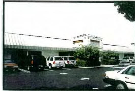
Administration Building 1500 Bollinger Canyon Road, San Ramon
