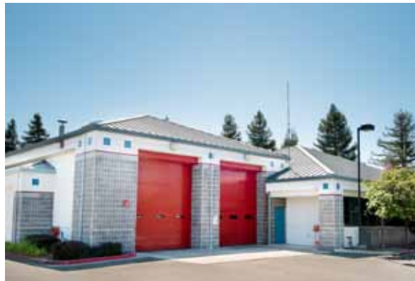
Station 38 1600 Bollinger Canyon Road San Ramon
