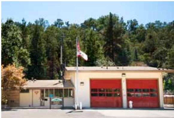
Station 32 1101 Stone Valley Road Alamo
