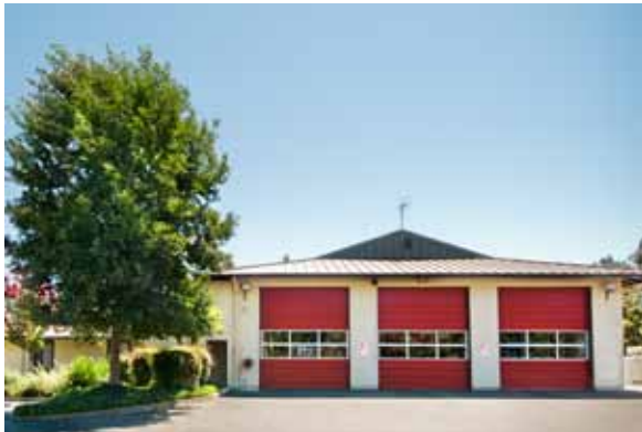
Station 34 12599 Alcosta Boulevard San Ramon
