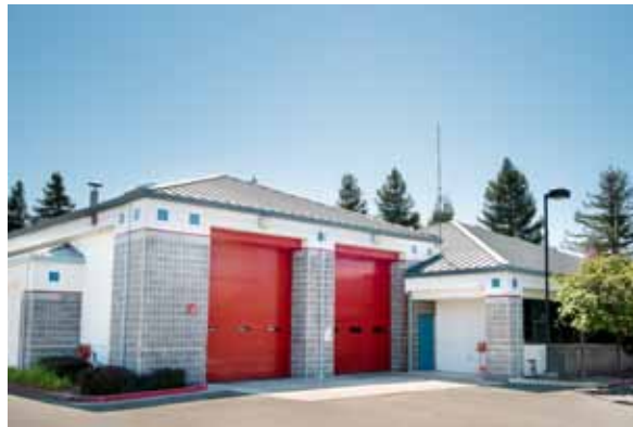
Station 38 1600 Bollinger Canyon Road San Ramon
