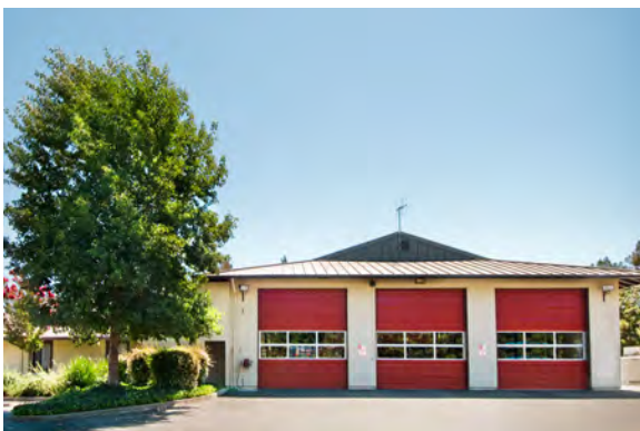
Station 34 12599 Alcosta Boulevard San Ramon
