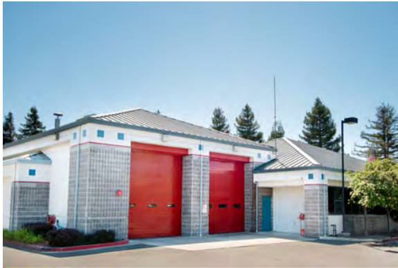
Station 38 1600 Bollinger Canyon Road San Ramon
