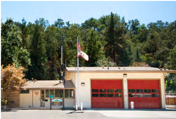
Station 32 1101 Stone Valley Road Alamo
