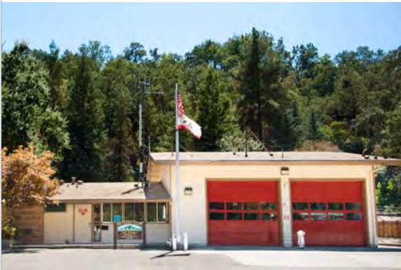
Station 32 1101 Stone Valley Road Alamo
