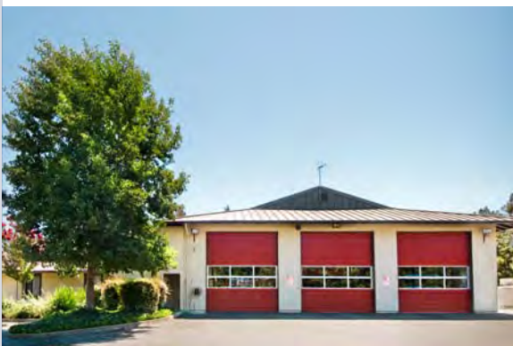
Station 34 12599 Alcosta Boulevard San Ramon
