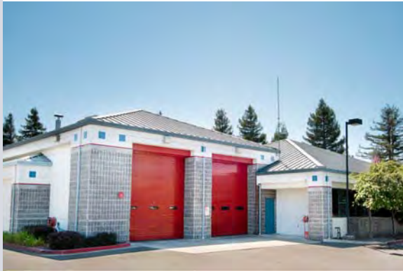
Station 38 1600 Bollinger Canyon Road San Ramon
