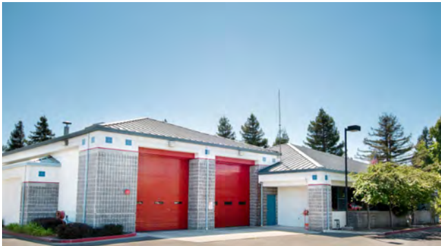
STATION 38 1600 BOLLINGER CANYON ROAD SAN RAMON
