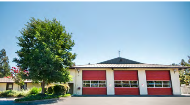
STATION 34 12599 ALCOSTA BLVD. SAN RAMON
