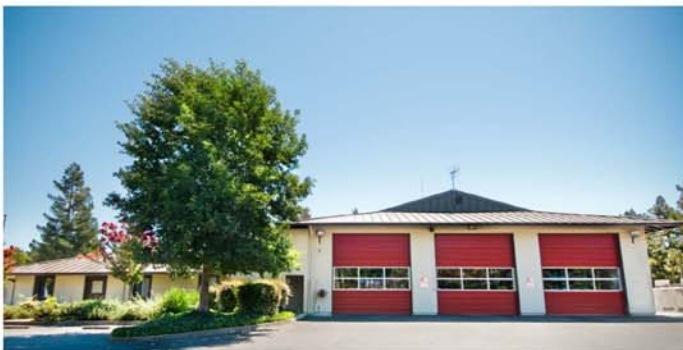
STATION 34 12599 ALCOSTA BLVD. SAN RAMON
