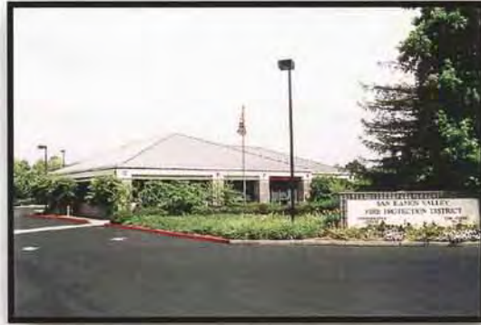
Station 38 1600 Bollinger Canyon Road, San Ramon
