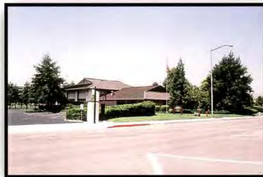
Station 34 12599 Alcosta Blvd., San Ramon
