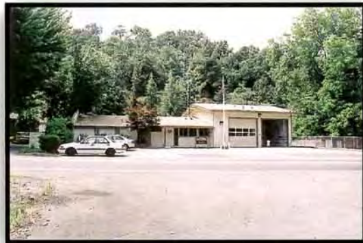
Station 32 1101 Stone Valley Road, Alamo
