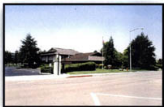
Station 34 12599 Alcosta Blvd., San Ramon
