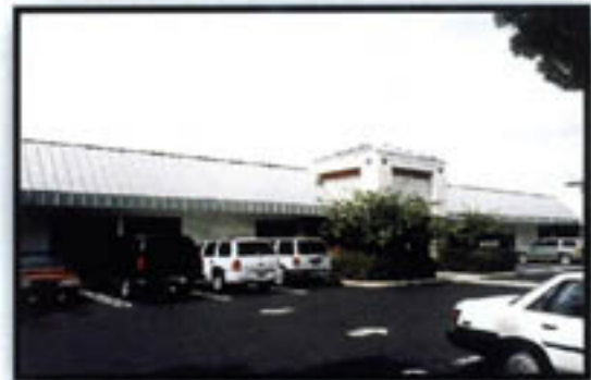
Administration Building 1500 Bollinger Canyon Road, San Ramon
