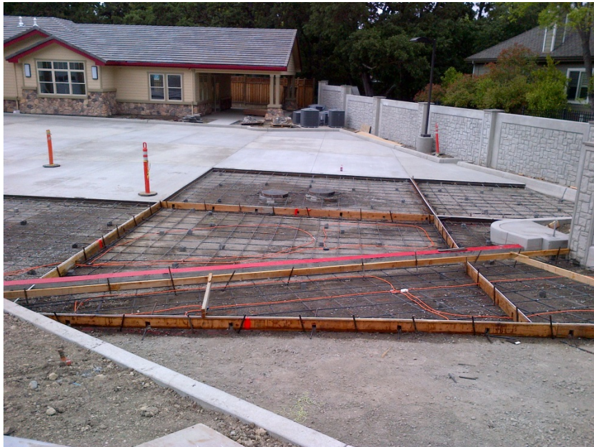
East parking lot
