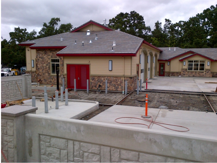
Fuel tank and parking area
